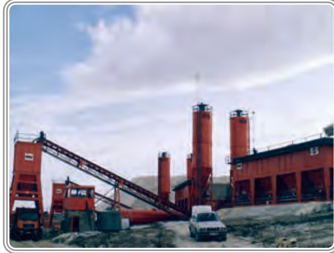
DOĐUŐ İNŐAAT / DROMEX ROAD & BRIDGE CONSTRUCTION ENTERPRISE 500 ton/saat MEKANİK STABİLİZASYON PLENTİ
